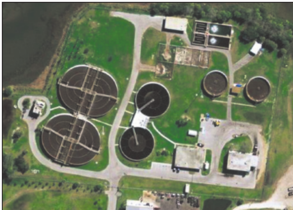
Figure 1: St. Augustine Wastewater Treatment Plant
